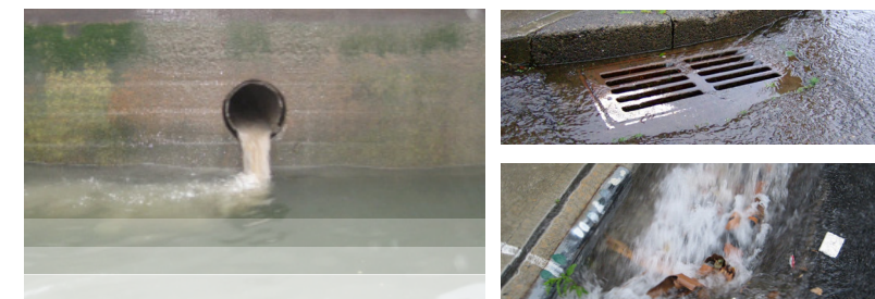
Below, left: combined sewer overflow is released into a local NJ waterway, right: top, stormwater rushes to a stormdrain and bottom, overflows
